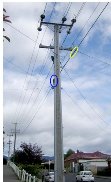
Figure 3: FlexNAP outside plant fibre distribution system- key FTTH enabler
